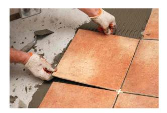
Wall and floor tiling refer to the laying of tiles of ceramics, mosaic and natural stone on walls, floors and staircases in houses, industrial and public buildings, Mosque, swimming pools, outside installations and facades to provide protective and decorative finishes. It also includes the construction of small walls and steps from bricks or blocks.
