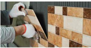
We then spread cement or adhesive with a trowel and lay the tiles in the desired pattern. We may have to cut tiles to fit around walls and obstacles. After the adhesive has dried, the joints between the tiles are filled with grouting cement. On large projects, Tile Fixture may work in teams. On smaller jobs, work alone.
